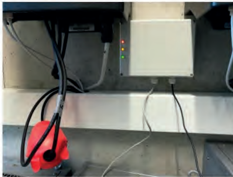
Figure 8 Online monitoring system in grey housing with traffic light display and cables for connection to the current transformer (grey wire) and the power supply (black wire) as well as the current transformer in red housing, installed on a DC cable between PV module and inverter
